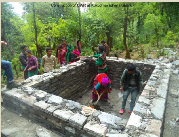
Construction of CWR at Kukudmayadhar (Kaemu)
